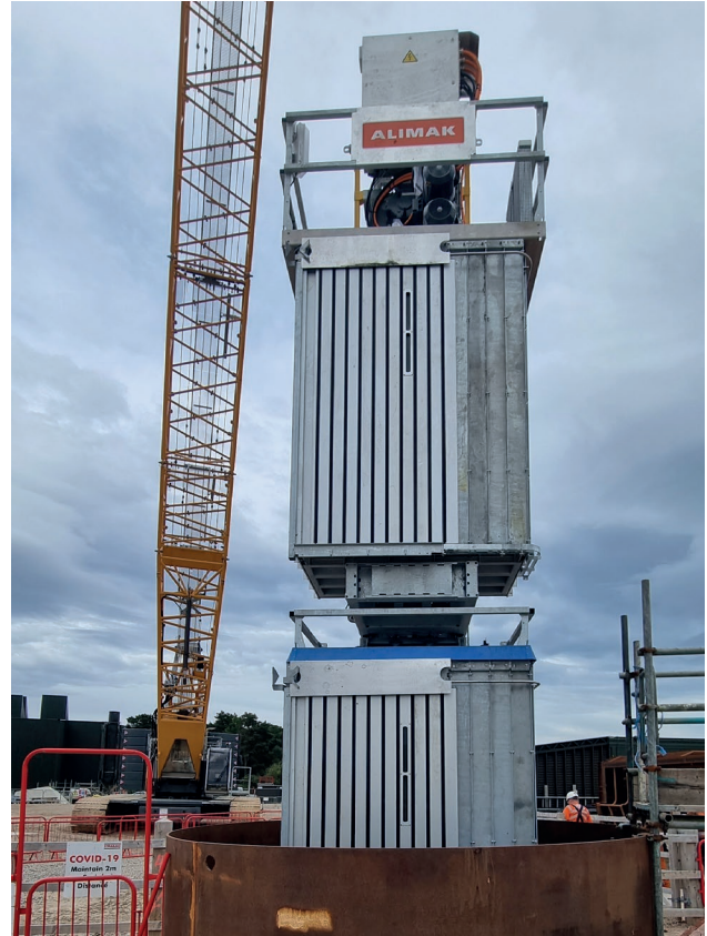
The custom "double deck" being installed into the shaft.
