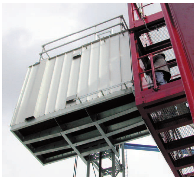
Bayer AG chemical plant, Dormagen, Germany
