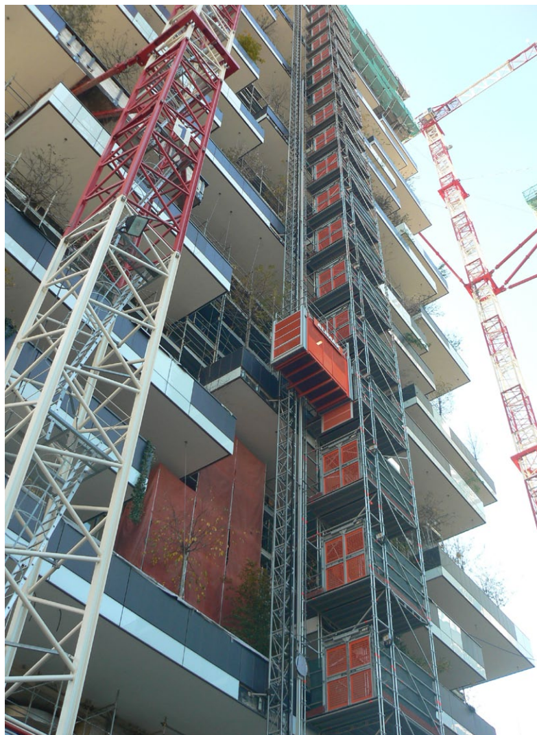
One of the Alimak hoists at work on the Bosco Verticale.
