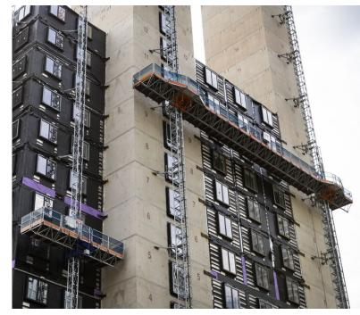
engineers added an extension to just one side of the hoist to allow the maximum car size of 4.45 m to fit within the space constraints.
