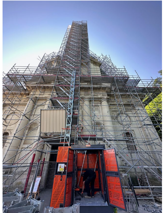
The new Alimak Medius 350 helps restore ancient chapel in Saumur, France.
