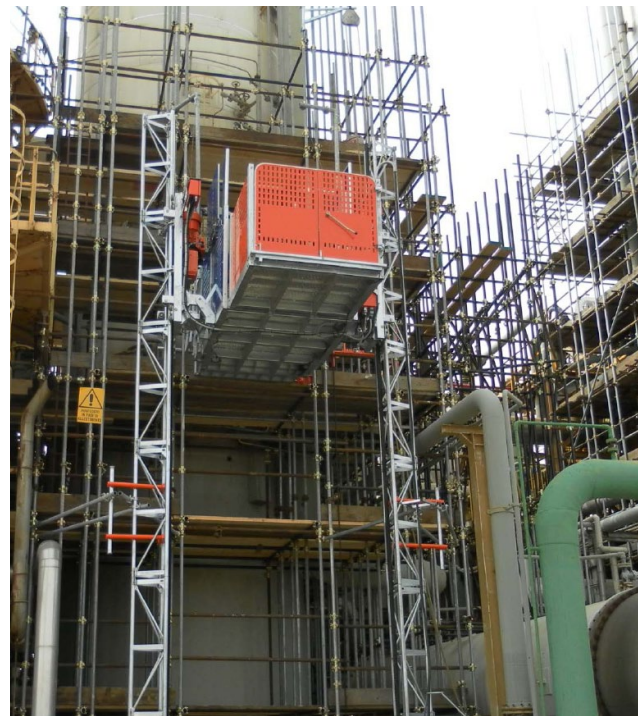
Alimak TPL speeds up scaffolding work at an industrial plant.
