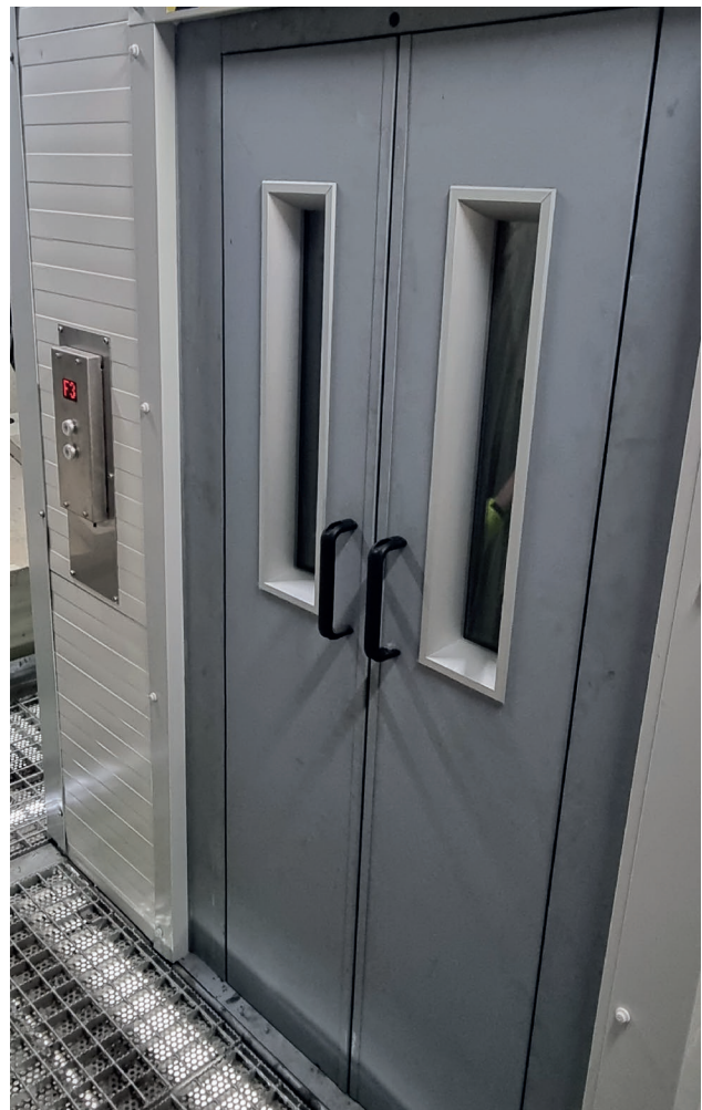
Bespoke landing doors were design due to limited opening space.
