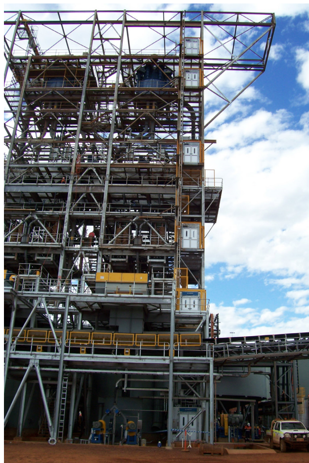
Christmas Creek Mine, WA, Australia
