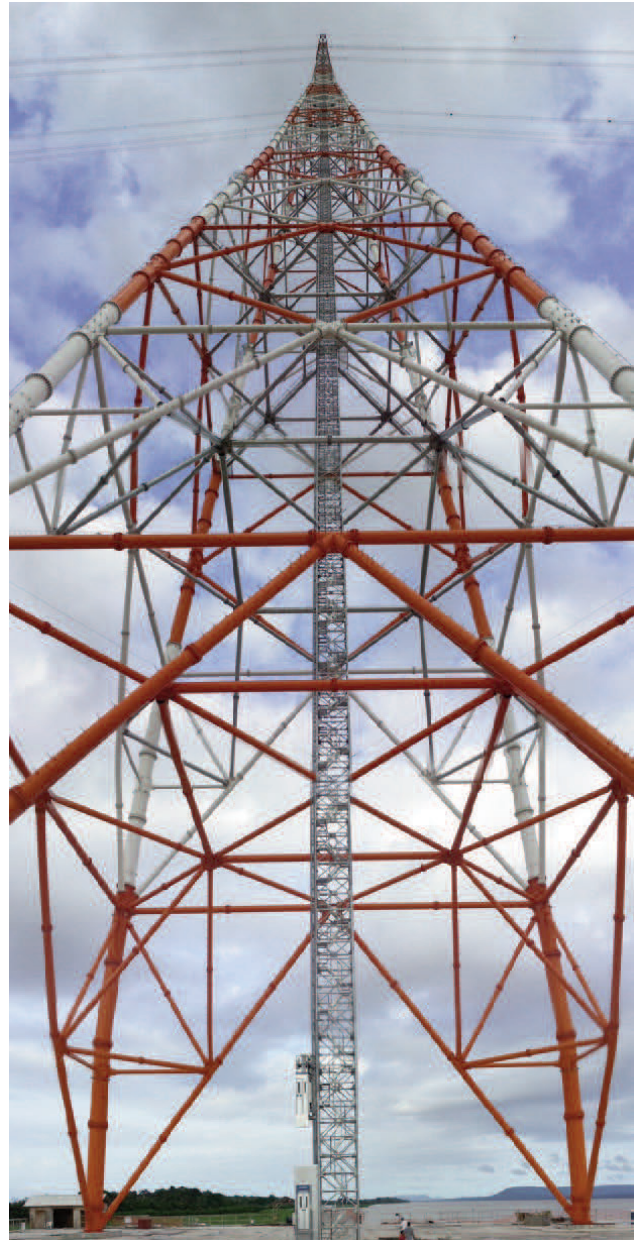
At heights of 295 metres, the transmission towers are the tallest of their kind in South America.
