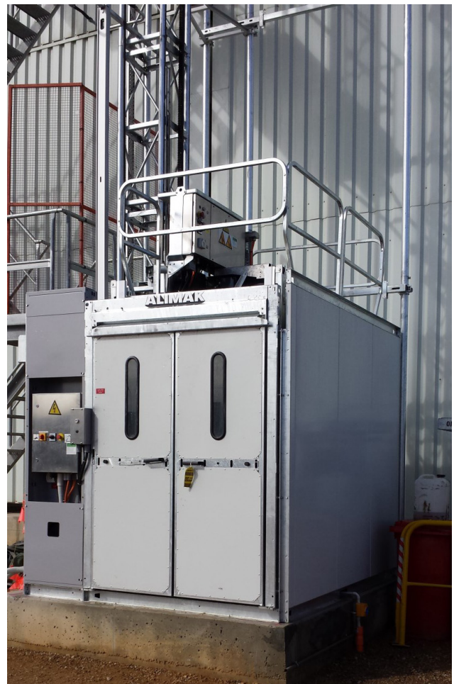
Wingfield Asphalt Manufacturing Plant, SA, Australia
