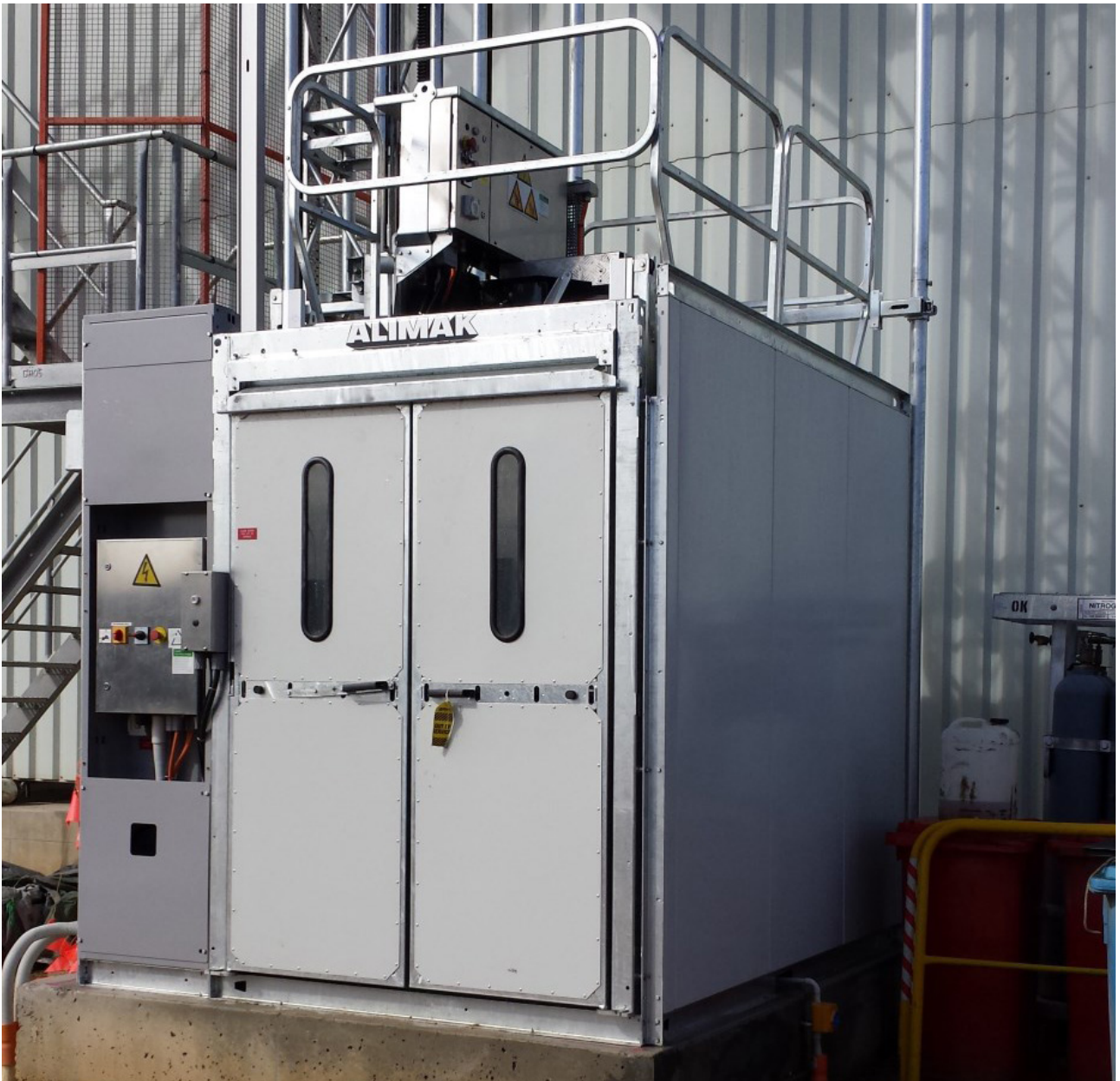
Wingfield Asphalt Manufacturing Plant, SA, Australia
