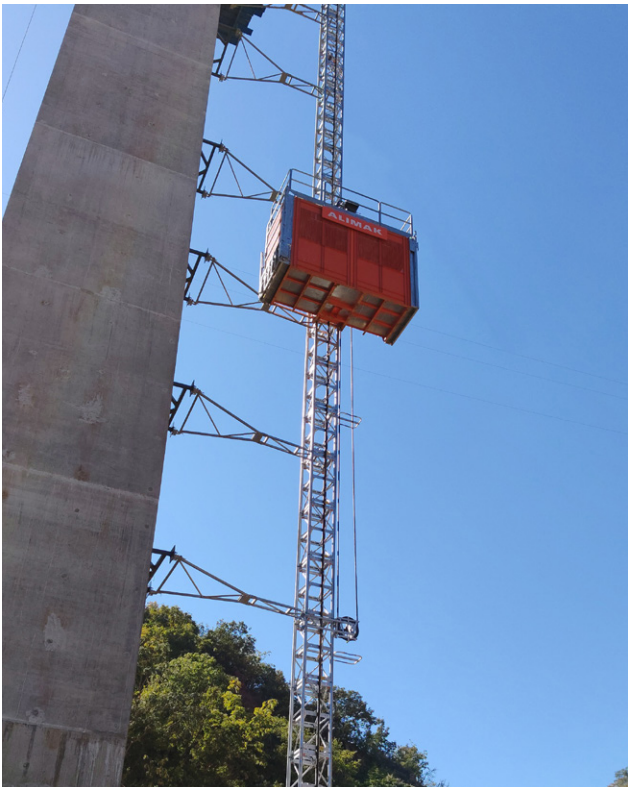
Alimak Levato 650 at Longchuan River Bridge project
