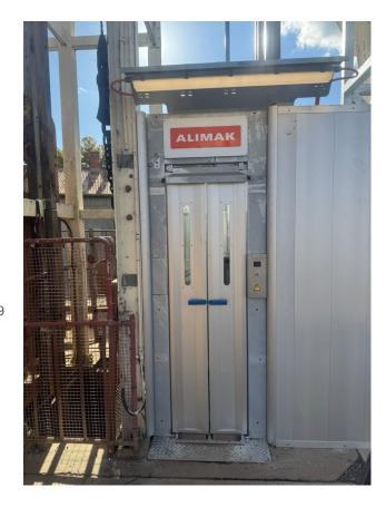
To avoid the high cost and complexity of crane hire — and to further enhance safety — Alimak introduced a permanent Tirak™ winch system with man-riding capabilities. This system now serves as both a materials hoist and an emergency recovery device, ensuring that workers have a safe and reliable means of evacuation in the event of an incident.
