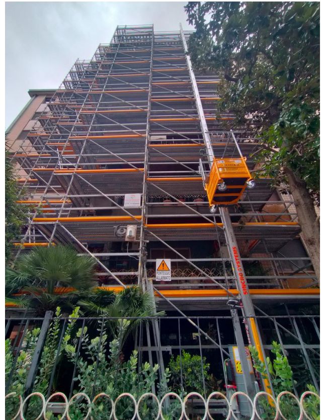
Alimak STS 300 supporting a scaffolding project in Cagliari.
