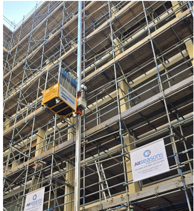
STS 300 supporting The Mark demolition project in London
